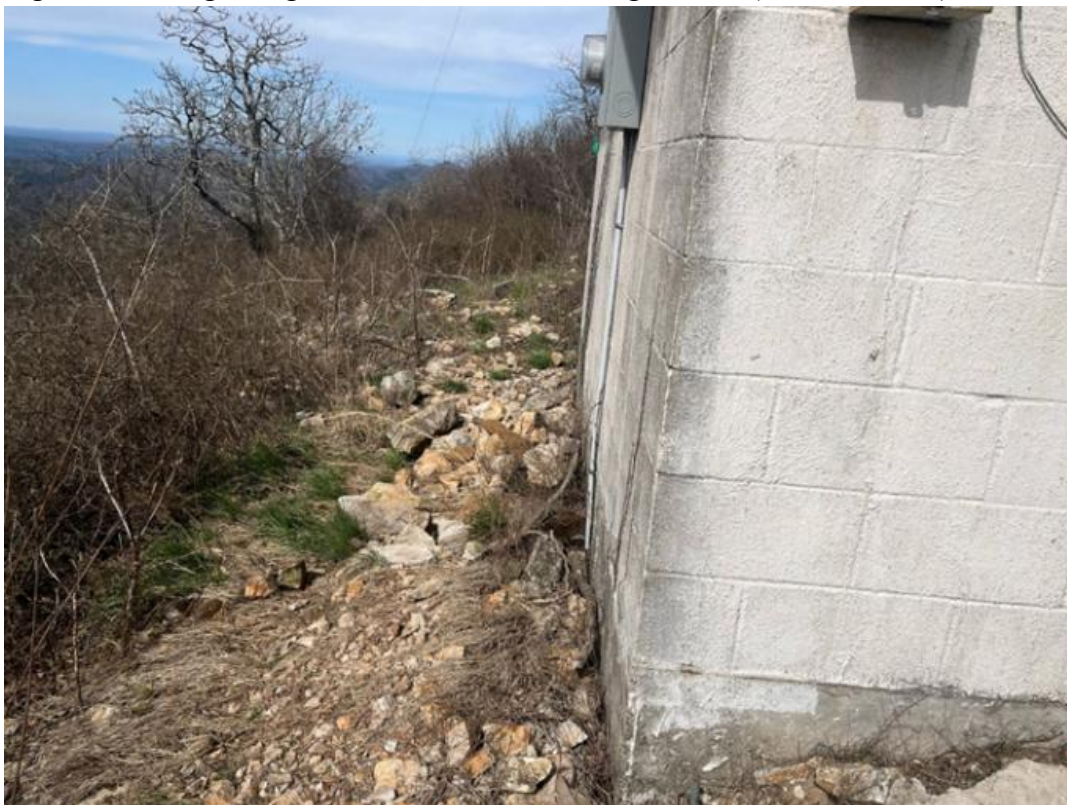
Figure B22: Degrading Foundation of Monitoring Shelter (sheer cliffside)
