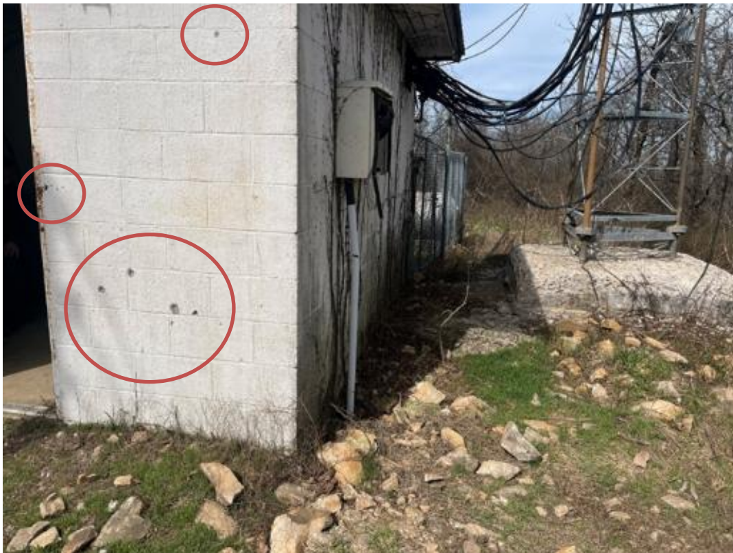
Figure B22: Degrading Foundation of Monitoring Shelter (sheer cliffside)
