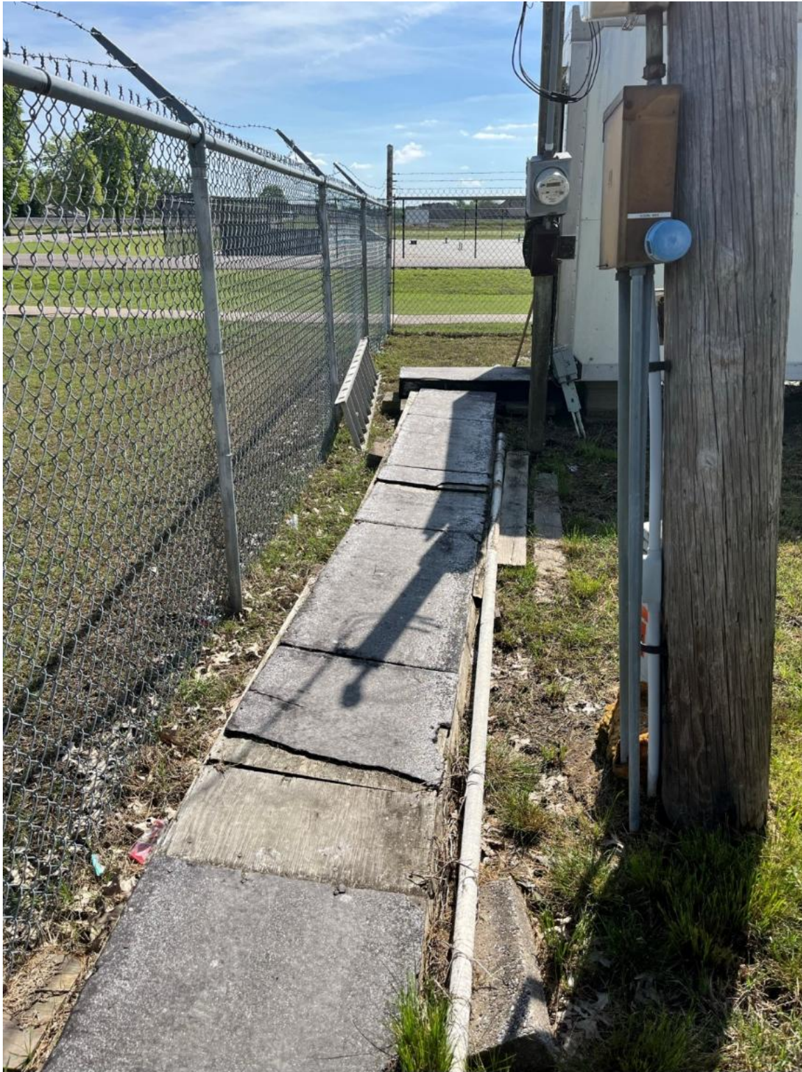
Figure B1: Current Marion Site, Exterior; Planks DEQ installed for traversing flooding conditions
