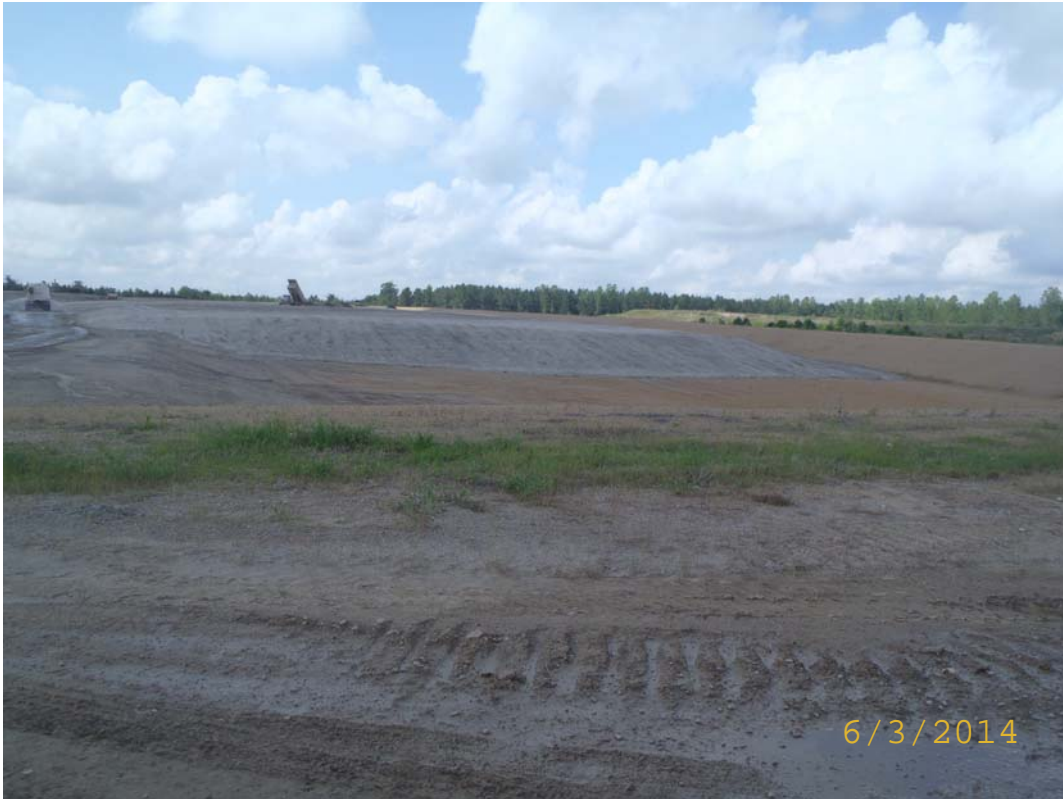
Permit #0311-S3N. Photo 1 and 2.
