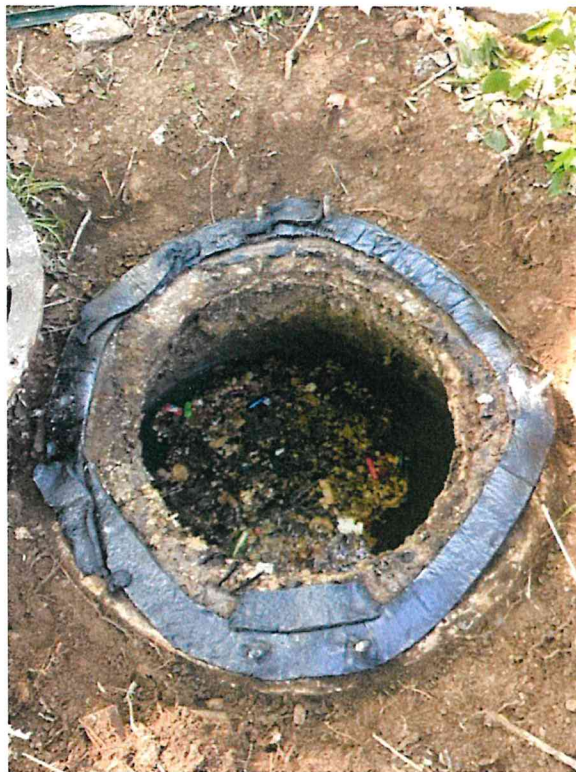
MH 12242 - After Ram-Nek replaced
