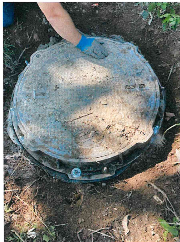
MH 12242 - New anchors installed, cover replaced
