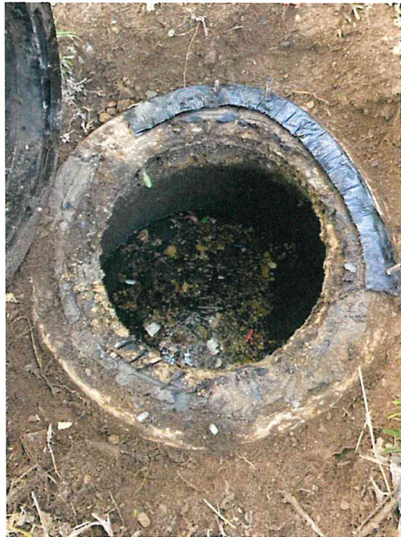
MH 12242 - Cover removed, during Ram-Nek replacement
