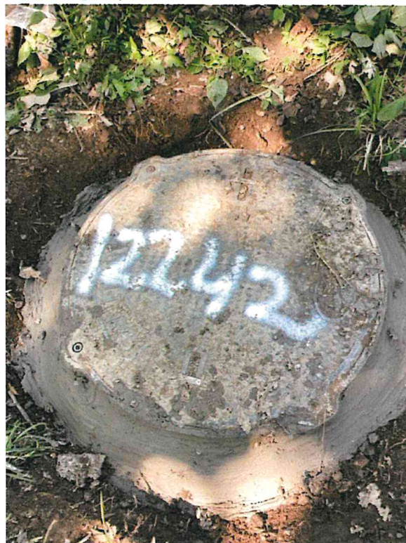
MH 12242 – Hydraulic cement seal
