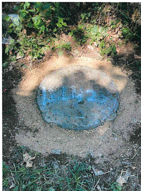
MH 12242 – Backfill around manhole
