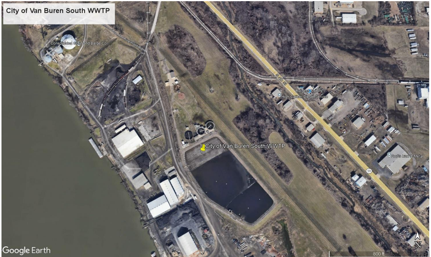
Figure 1. An aerial view of The City of Van Buren South WWTP.
