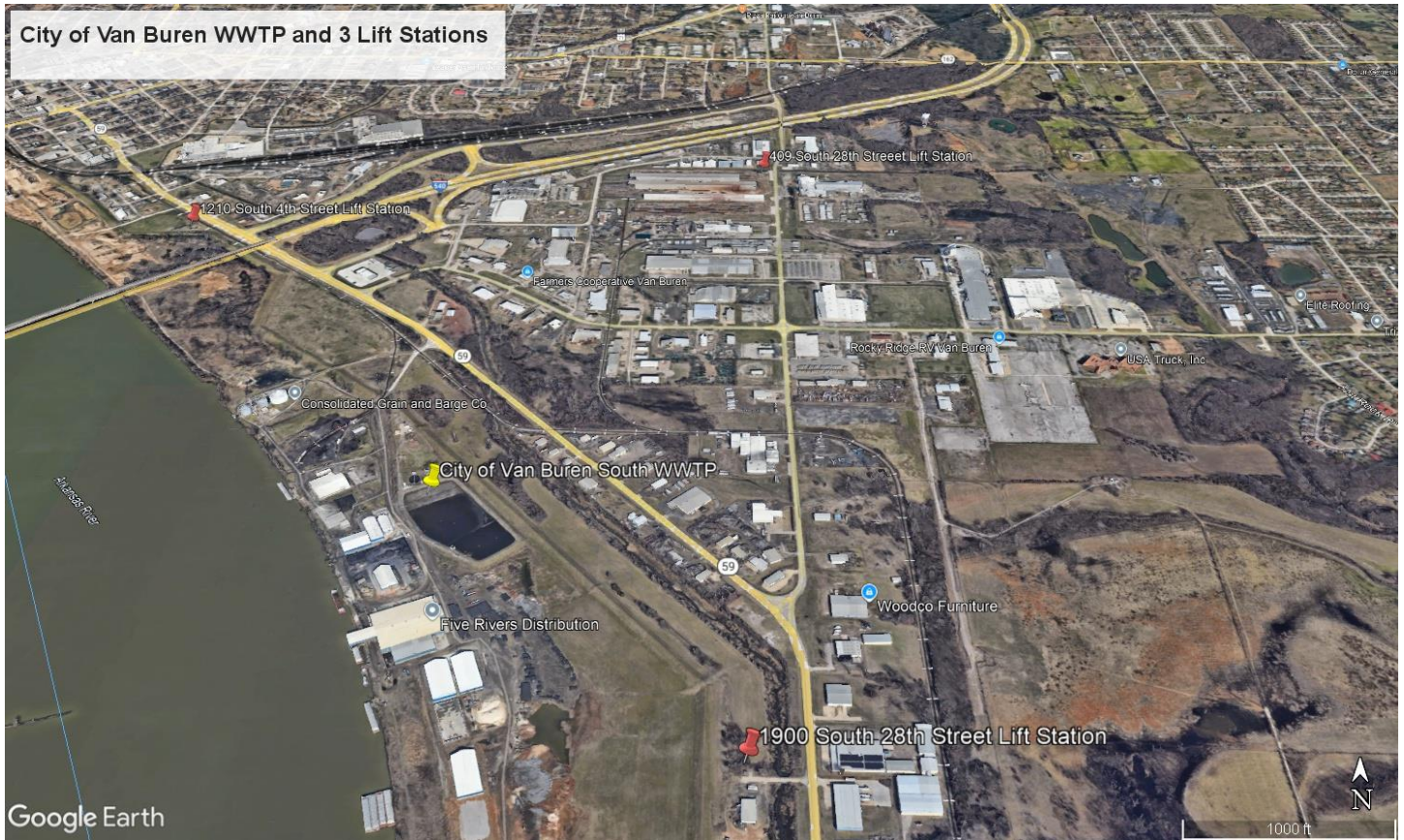
Figure 1. An aerial view of The City of Van Buren South WWTP and 3 Lift Stations.
