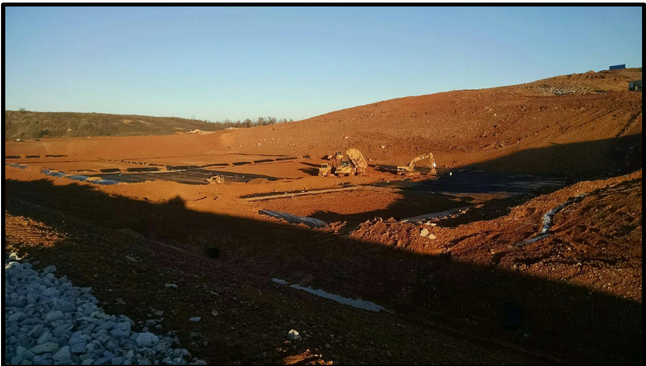
8. Looking west at completed rainflap berms and placement of protective cover..
