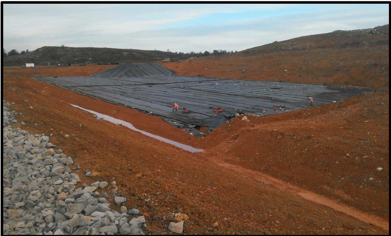
6. Looking west at completed double-sided geocomposite deployment
