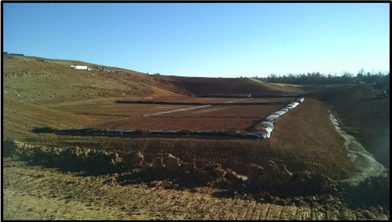
9. Looking east at completed Cell B2.
