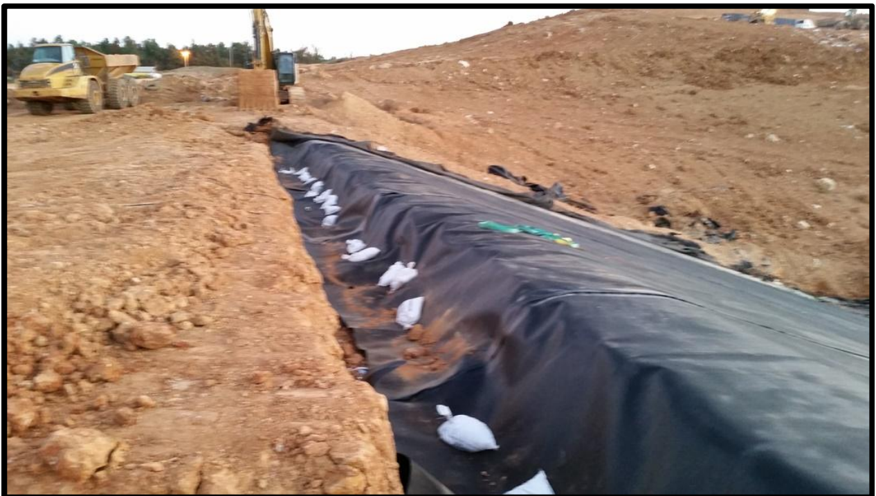
4. Looking north at 60 mil geomembrane in the west anchor trench.
