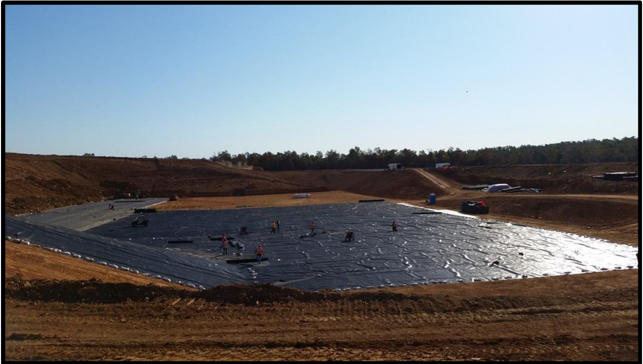
3. Looking east at deployment and seaming of 60 mil textured geomembrane..
