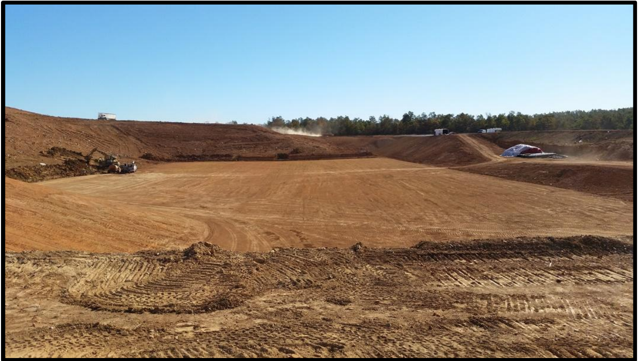
1. Looking east at top of subgrade.
