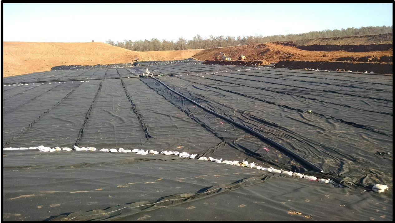
7. Looking east at 6" HDPE leachate line and placement of the rainflap berm.
