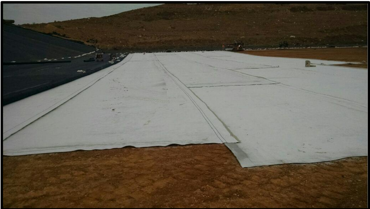
2. Looking north at deployment of geosynthetic clay liner (GCL).
