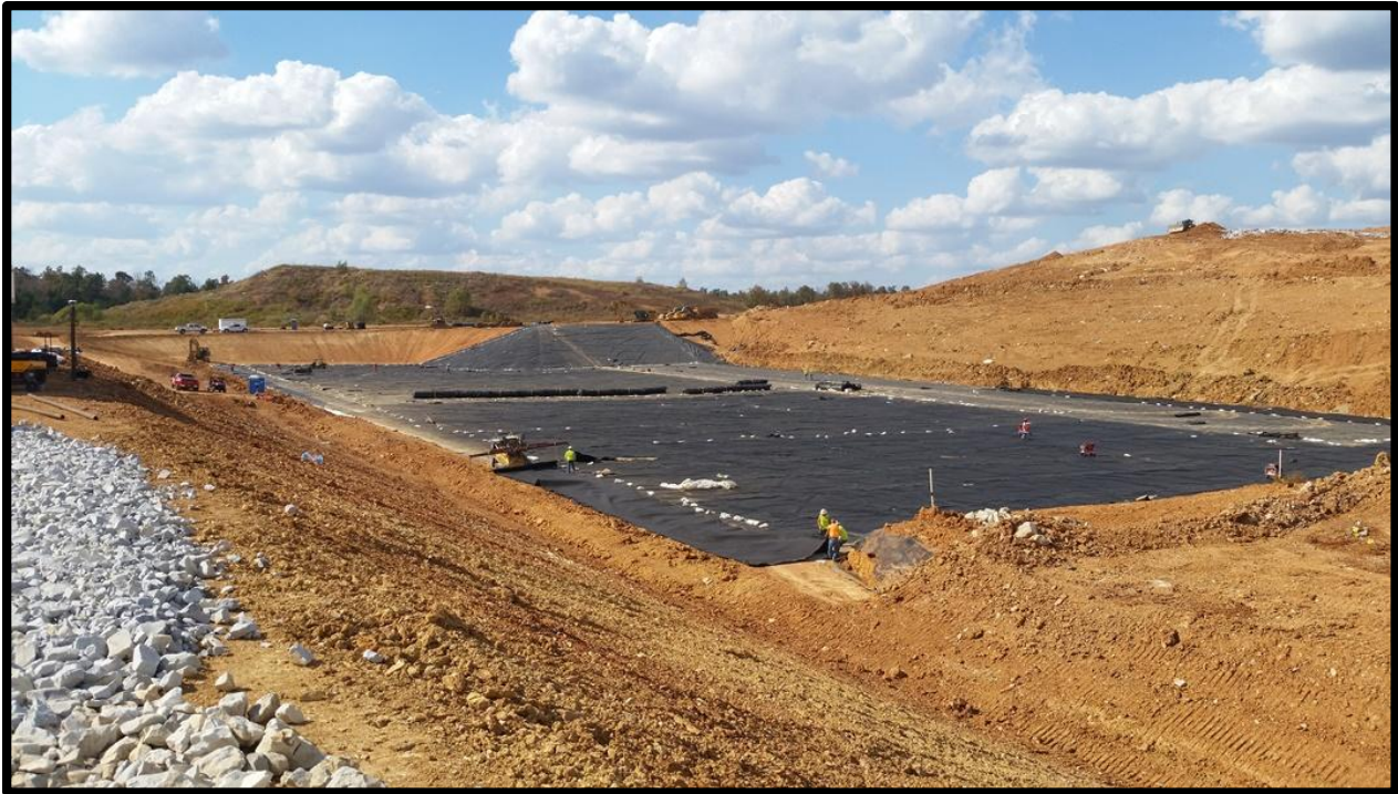
5. Looking west at completed 60 mil geomembrane and deployment of double-sided geocomposite.
