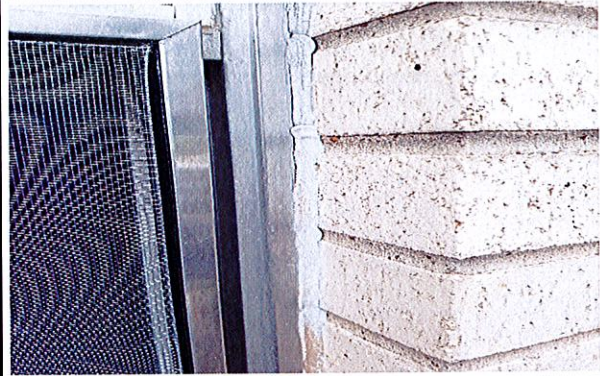
4771-02-03 & 04: Perimeter Window Caulk
