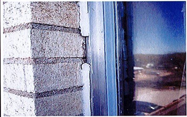
4774-11-21 & 22: White Perimeter Window Caulk
