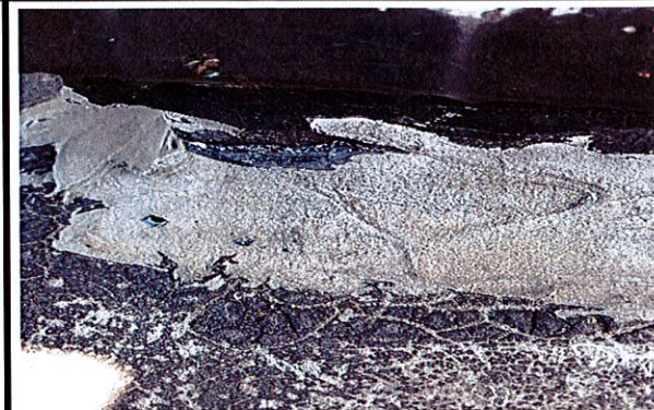
477R-04-04: Middle Roof - Penetration Mastic - 15% Chrysotile
