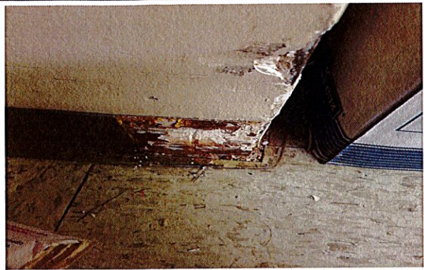
4771-21-41 & 42: Gray Cove Base & Mastic
