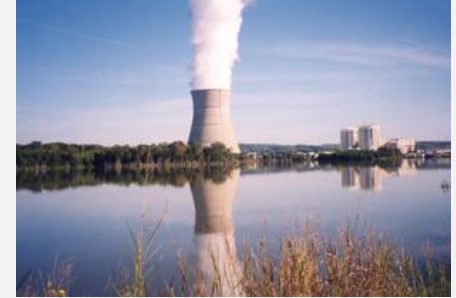
Industrial Water Supply
